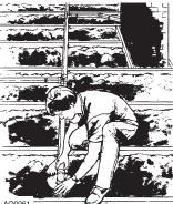
When you are satisfied that all fittings and tubing are aligned for maximum air flow, make sure that all your cuts are square and that all joints are tight. Then, prepare the tubing and cement the joints as described in "Working With Plastic Tubing," page 5.
