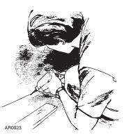
Once you've found the location in the partition wall, you must center the access hole in the middle of the wall. Measure half the thickness of the wall and mark the center of the wall where you will drill the access hole. If you cannot see the plate, you can determine this measurement from upstairs. At the nearest doorway, measure the thickness of the wall, including the baseboard.
