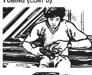
Tuck the 6" wire lead inside the flexible tubing so that it will not snag inside the wall.
