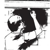
Attach the tubing to the joists or ceiling with either perforated metal or support strapping (support strapping is available from NuTone).
