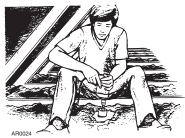
Now, use a flashlight to inspect the wall cavity through the access hole. Make sure no hidden obstacles will interfere with the tube installation. (If this inspection reveals an obstacle, find a new inlet location.) Repeat this procedure in your attic or basement until your access holes are drilled.
