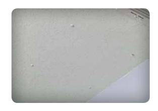
**3.** From below, place the cut-out template on the ceiling at each location, making sure that you have at least 2 inches of clearance all around it. While holding the template in place, mark its outline with a pencil.
